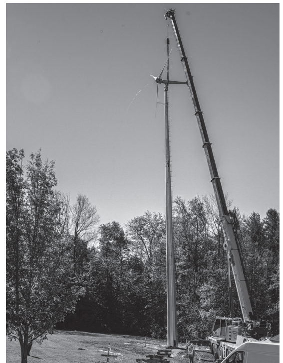
Wind Turbine installation, photo by Art Alpert
